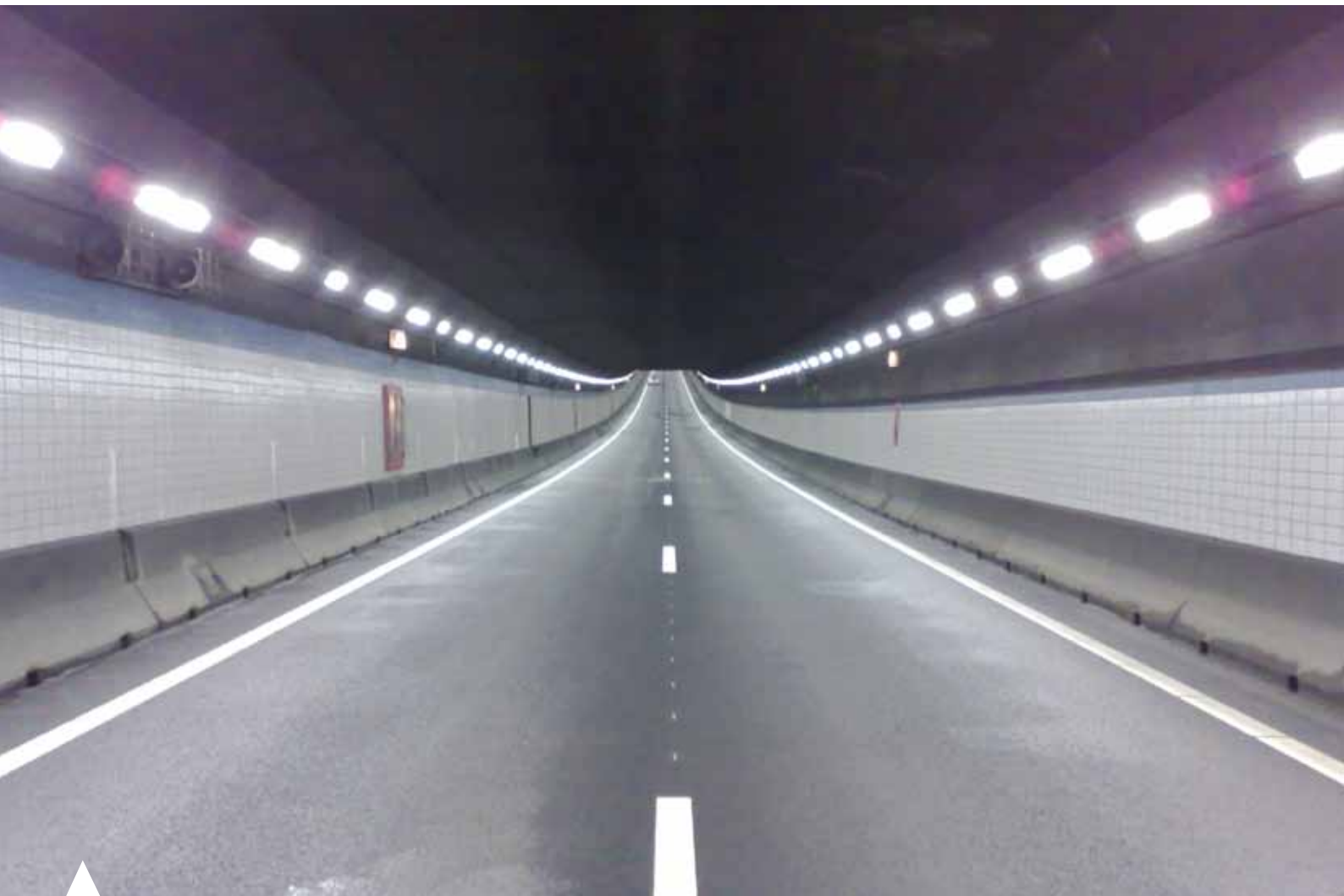
Coentunnel, Amsterdam, The Netherlands
