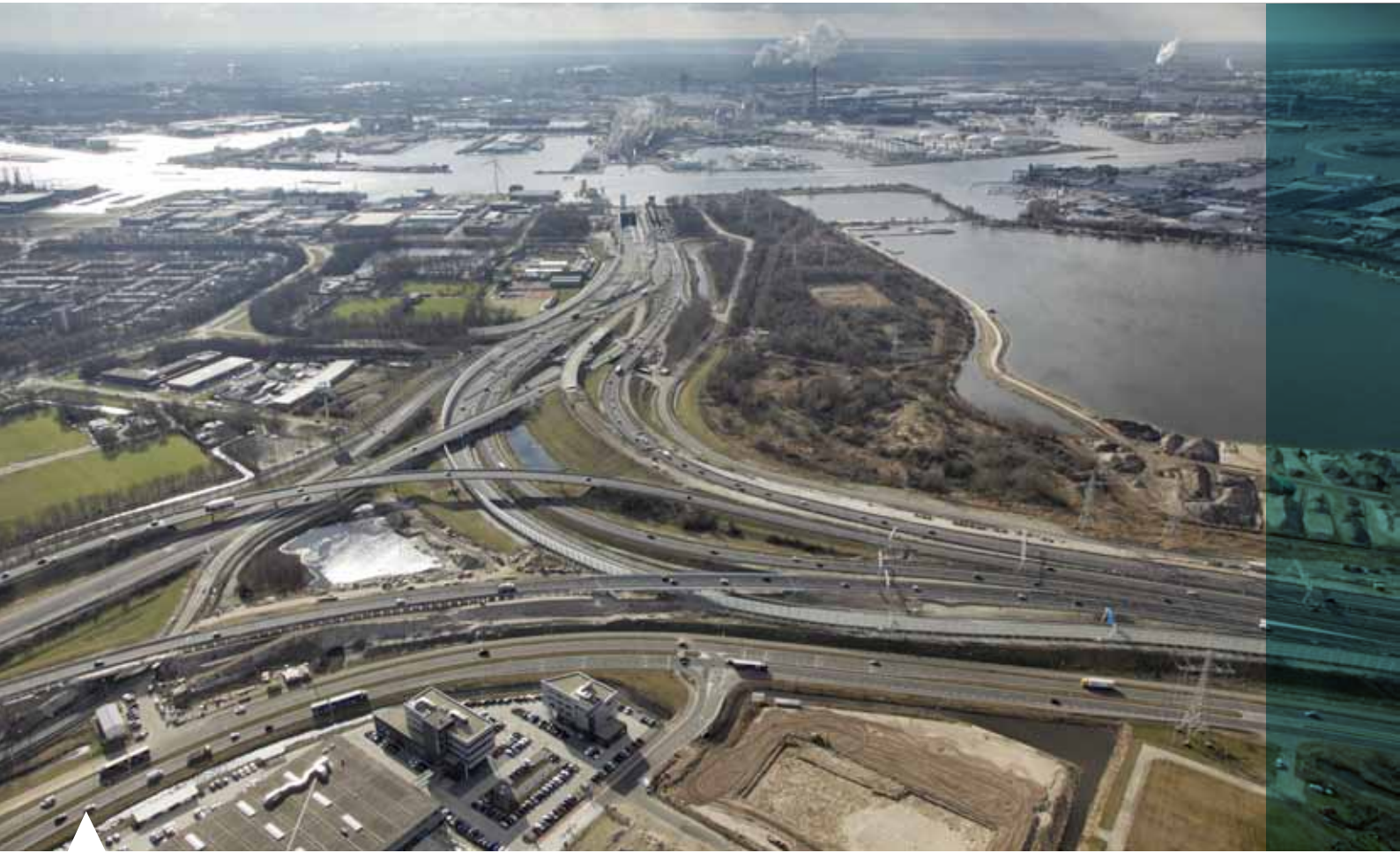
Coentunnel, Amsterdam, The Netherlands
