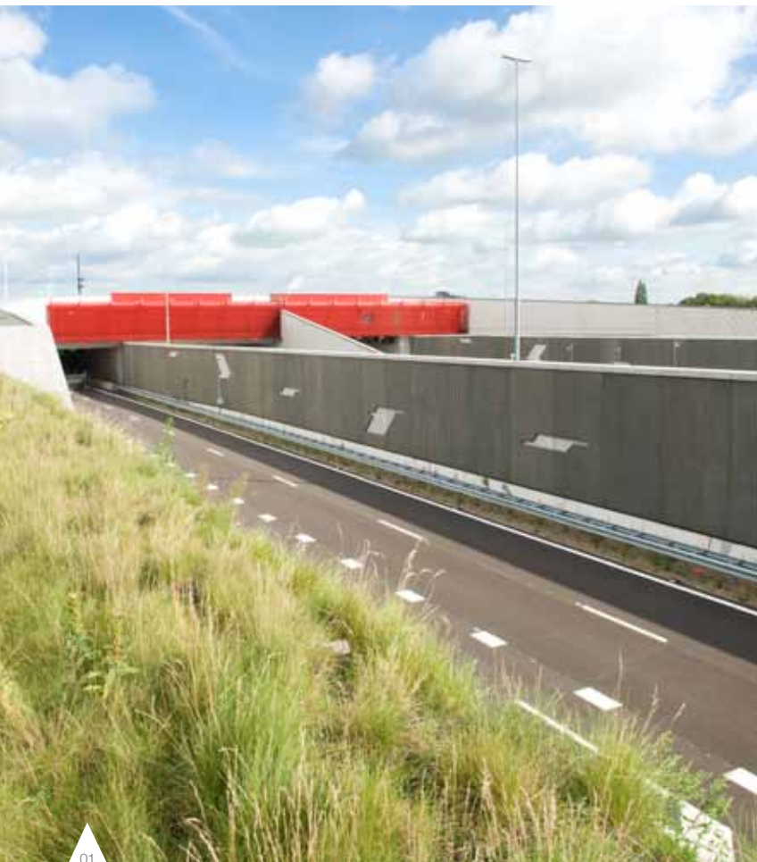
01 DODO Tunnel, Utrecht, The Netherlands
