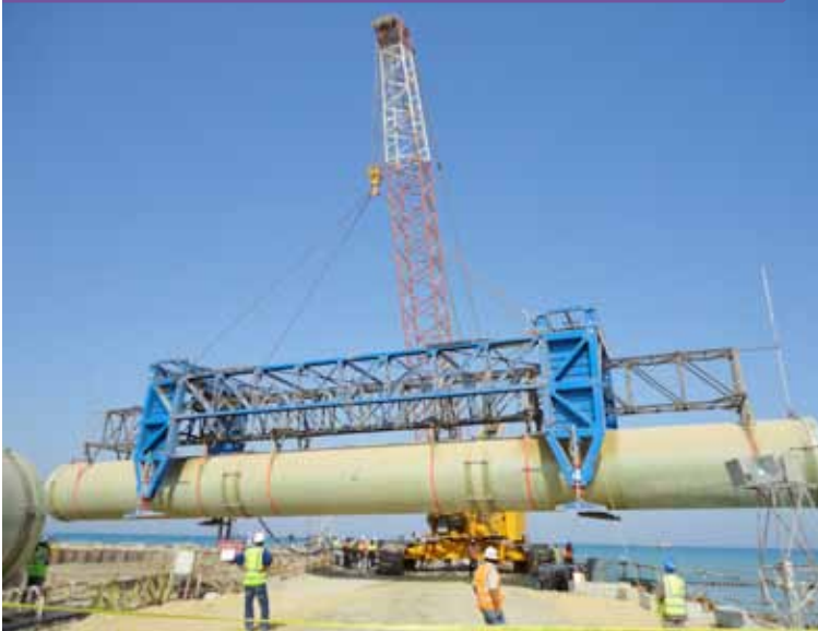
01 Wheatstone LNG Project, Onslow, Australia
