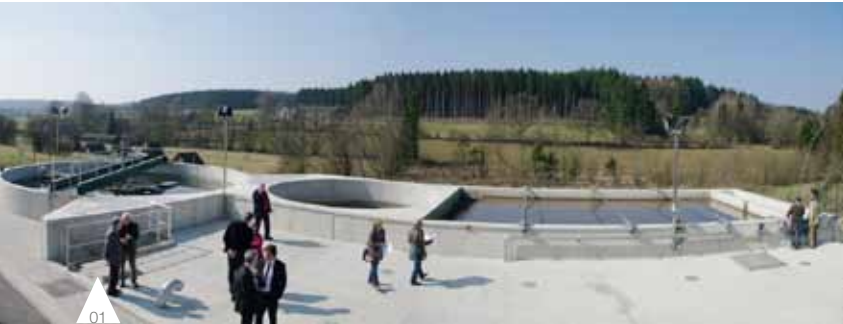
01 Biological Treatment Plant, Paliseul, Belgium
